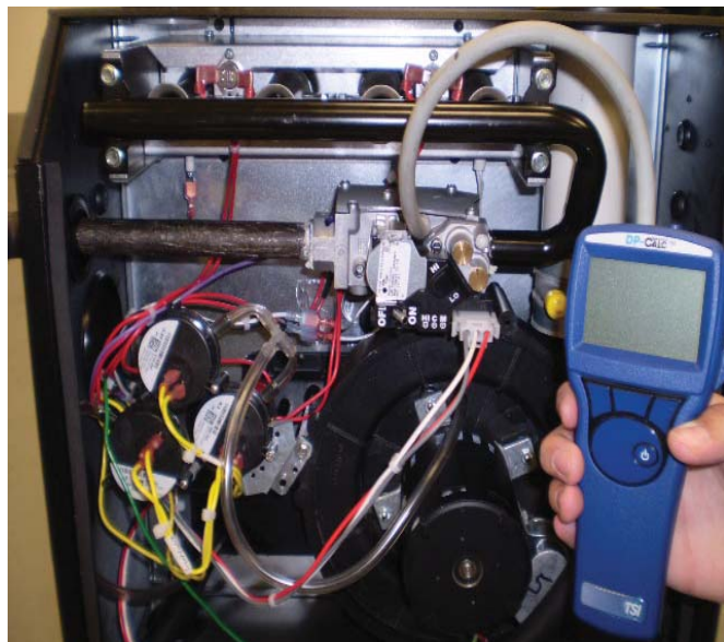
FIGURE 30 - MANOMETER MEASURING GAS MANIFOLD PRESSURE
