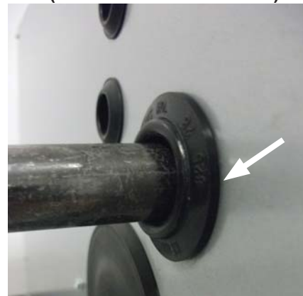
FIGURE 27 - FURNACE GAS PIPE CONNECTIONS (NOTE RUBBER GROMMET)
