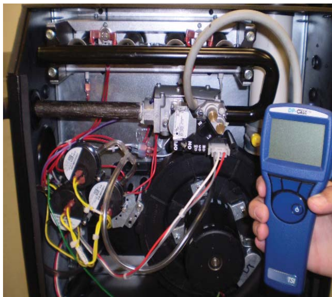
FIGURE 30 - MANOMETER MEASURING GAS MANIFOLD PRESSURE
