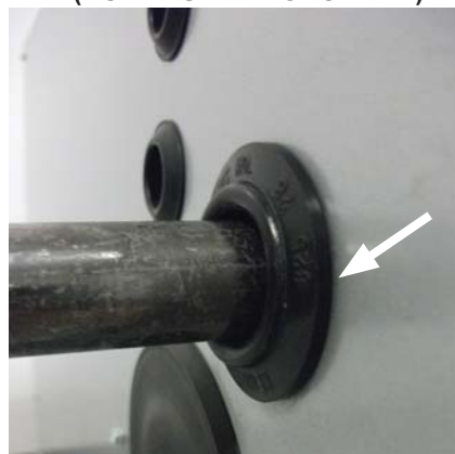
FIGURE 27 - FURNACE GAS PIPE CONNECTIONS (NOTE RUBBER GROMMET)
