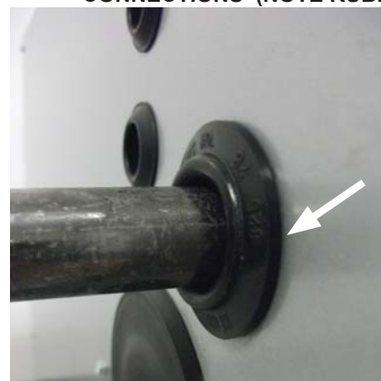
FIGURE 28 - FURNACE GAS PIPE CONNECTIONS (NOTE RUBBER
