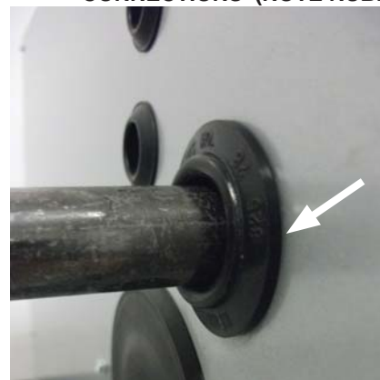
FIGURE 28 - FURNACE GAS PIPE CONNECTIONS (NOTE RUBBER
