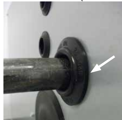
FIGURE 28 - FURNACE GAS PIPE CONNECTIONS (NOTE RUBBER
