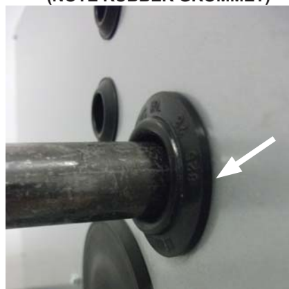
FIGURE 27 - FURNACE GAS PIPE CONNECTIONS (NOTE RUBBER GROMMET)
