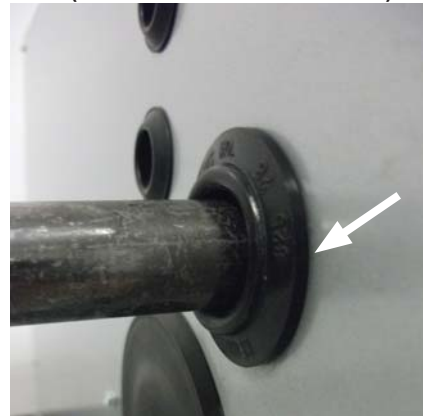
FIGURE 27 - FURNACE GAS PIPE CONNECTIONS (NOTE RUBBER GROMMET)
