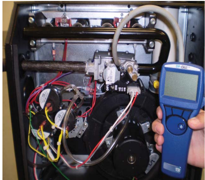
FIGURE 30 - MANOMETER MEASURING GAS MANIFOLD PRESSURE
