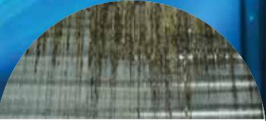
Even a minimum coil biofilm build up of debris 0.042 inches thick (imagine plastic wrap) will substantially **decrease system efficiency and performance by over 20 to 30 percent.**
